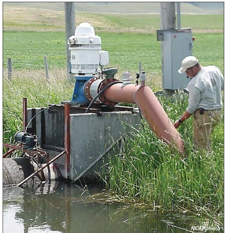
option. Running an oversized pump with a mainline valve half-closed is like driving a car with your foot on the brake and the accelerator at the same time.
